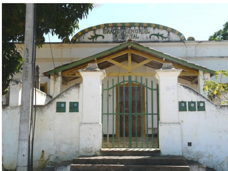
Figura 3 –Entrada principal do Grace Memorial Hospital
